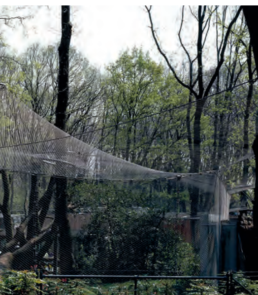
Enclosure construction in an existing forest; tree trunk passages integrated in the roof mesh
