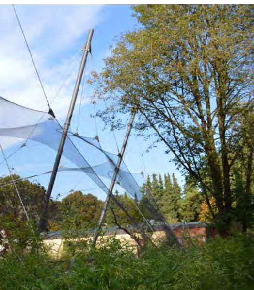
Walk-in aviary for wading birds with exterior tensioning cable construction
